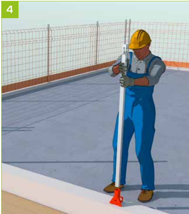
- Install the posts.
