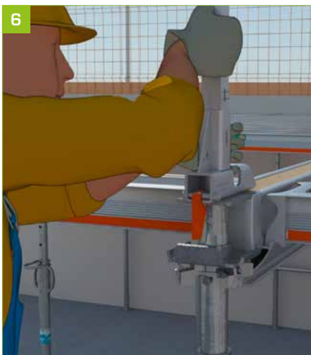
- The post anti-dropout system locks automatically onto the adapter.
