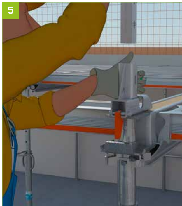
- Fit the AlphiSafe post in the adapter.
