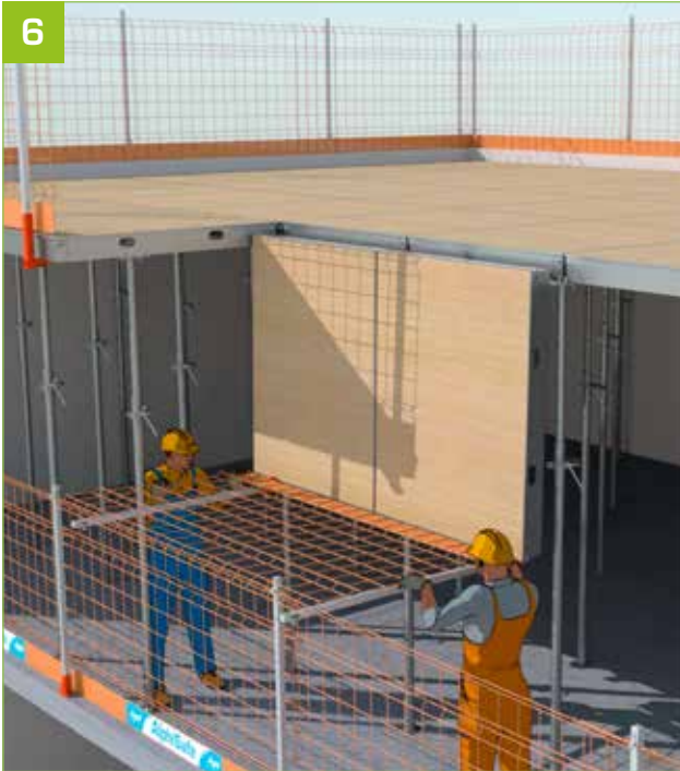
- Install the AlphaSafe mesh.
