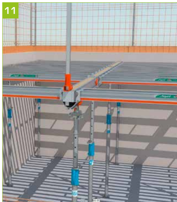
- Continue to install the formwork using this method.
