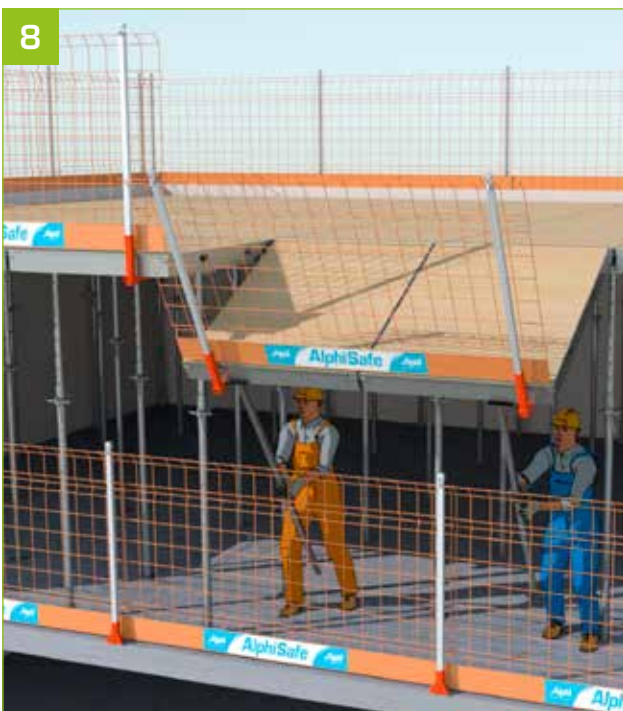
- Lift the panels using the MaxiDalle poles.
