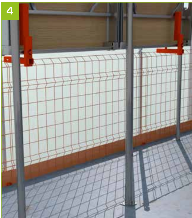
4 - To the rear of the panels, at their ends, mount 2 AlphiSafe MaxiDalle adapters.
