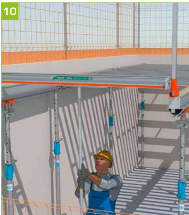
- Follow the same procedure with another primary beam and install a secondary beam at their ends using the TopPerche.
