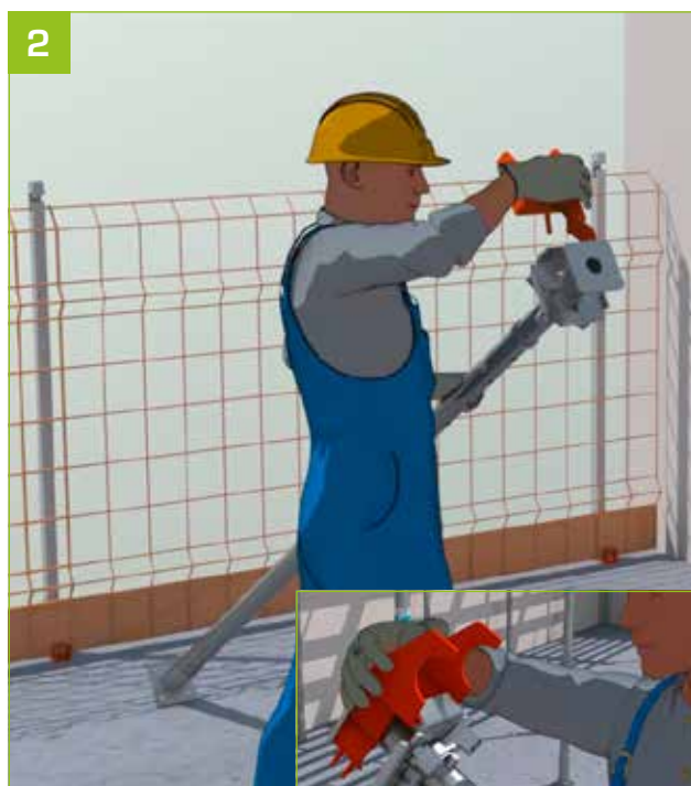
- On the ground, place the new-generation bracket on the technical support (or the insulated head) that is to receive the primary beam in a cantilever configuration.
