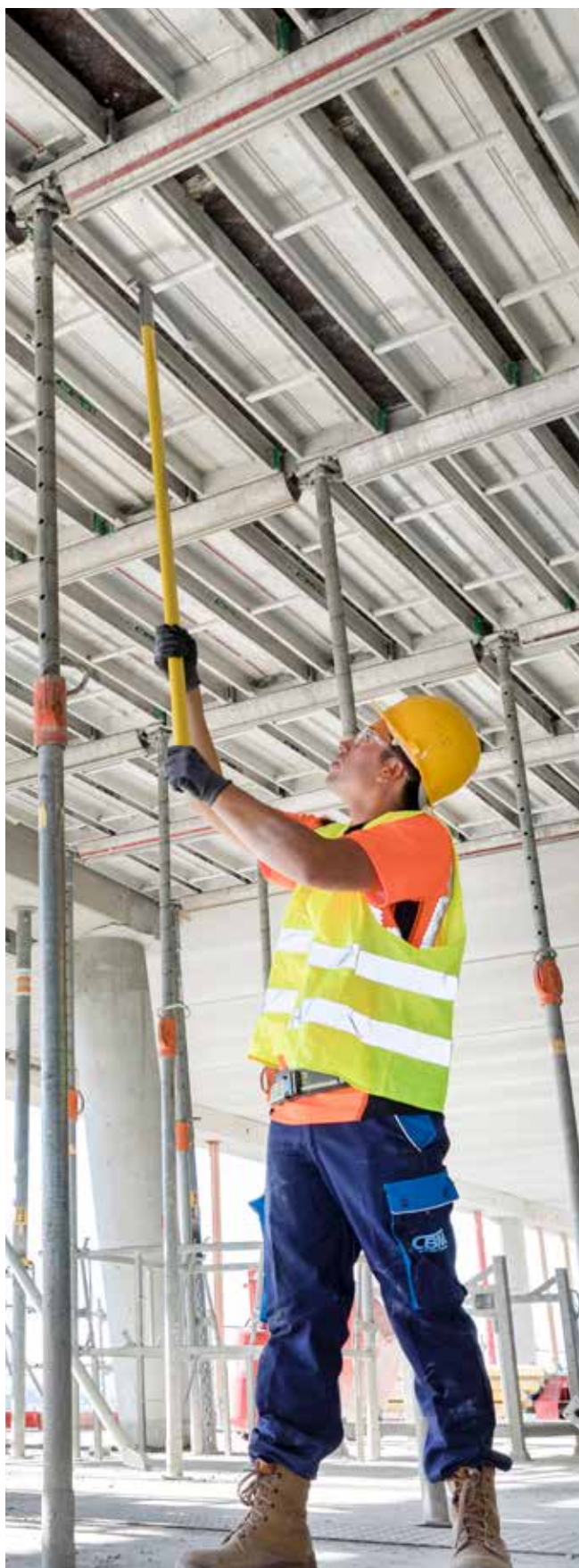
Long-range form stripping tool in use
