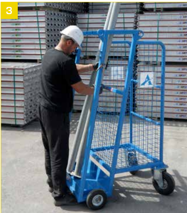
- Positioning props in the trolley.
