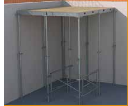
- A cross-member frame is fitted provisionally on the first 4 props.
