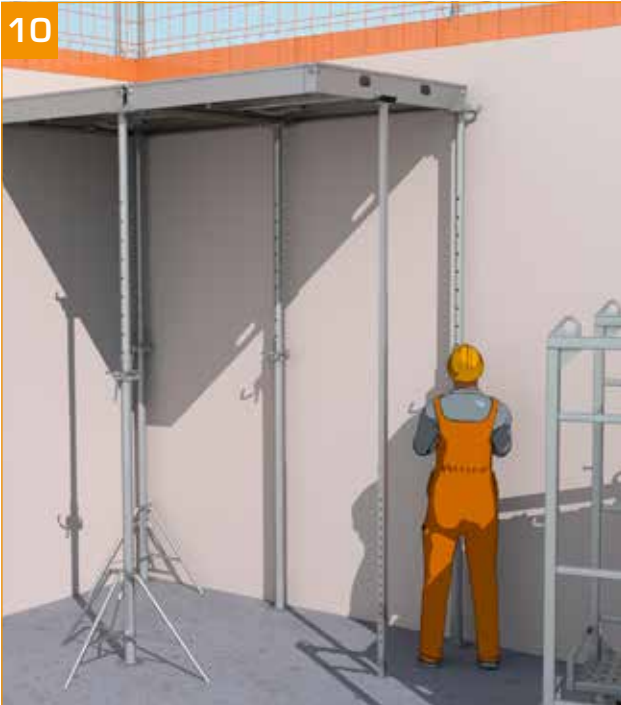
- Position the final 2 props under the panel.
