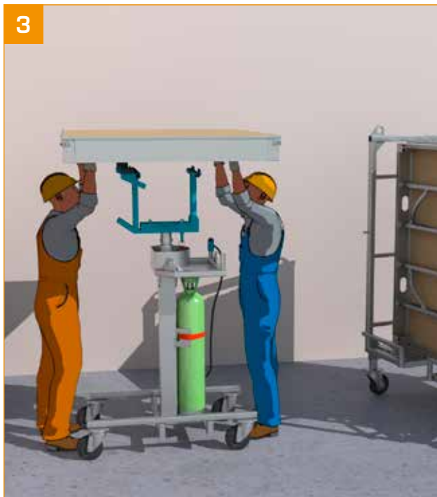
3 - The first panel is placed flat and centred on the head of the device.
